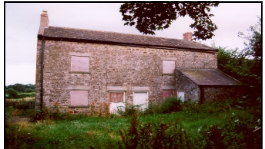
Everywhere there was evidence of vandalism - Hipswell Mill October 1998
