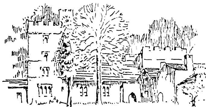
Nappa Hall from the south
